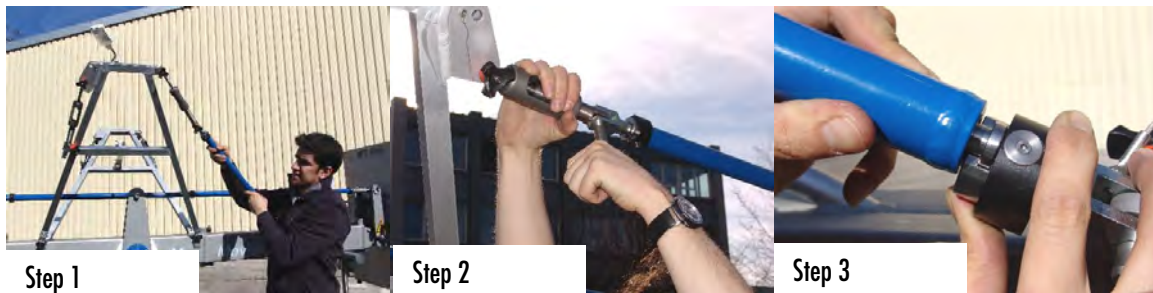
Fig. 38: Mounting the strut bar and adjusting the length
