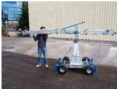
Fig. 17: Mounting the front crane elements
